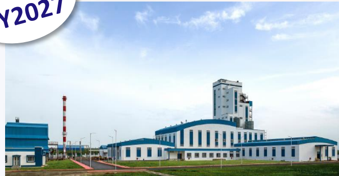
Expansion of India spray-dried soluble coffee manufacturing facility
