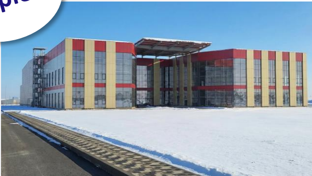
Completed coffee mix manufacturing facility in Kazakhstan
