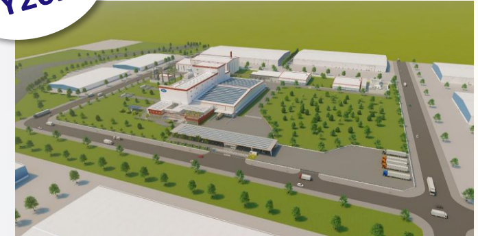
New freeze-dried soluble coffee manufacturing facility in Vietnam
